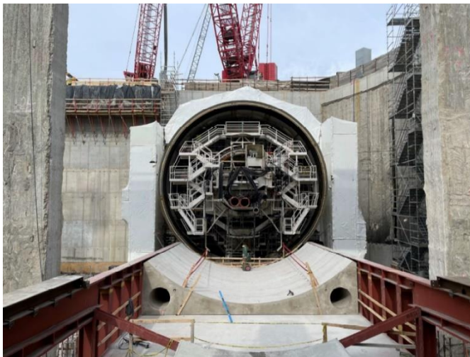
◀ South Island TBM Shield and Gantry Cradle
