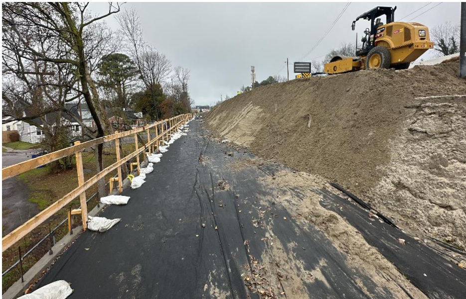
◀ I-64 EB (Segment 3) Placing embankment at Retaining Wall 311
