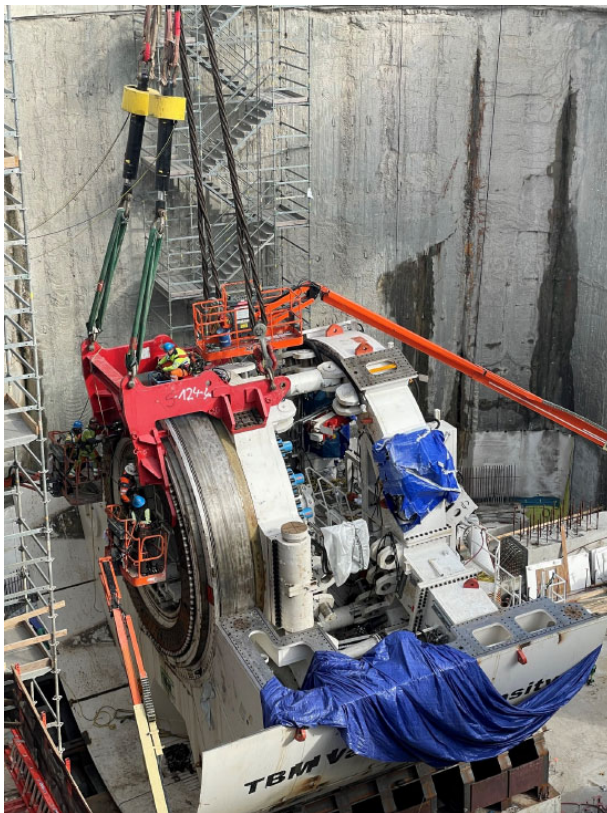
◀ South Island TBM main drive installation
