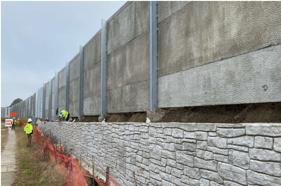
◀ I-64 EB (Segment 4) Sound wall 4-6 and retaining wall 405A below
