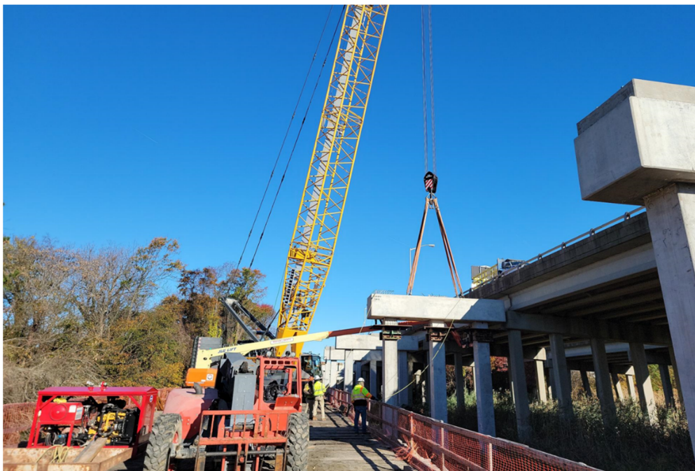
◀ Bay Avenue Bridge Setting Bent 9 precast cap for eastbound widening.
