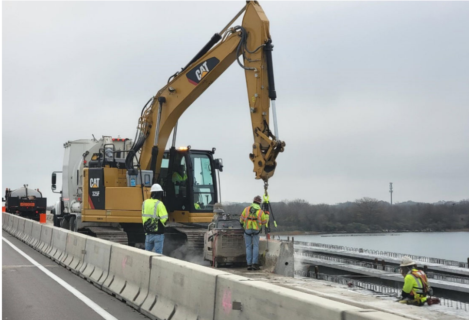
◀ Willoughby Bay Bridge Eastbound parapet wall removal for widening work
