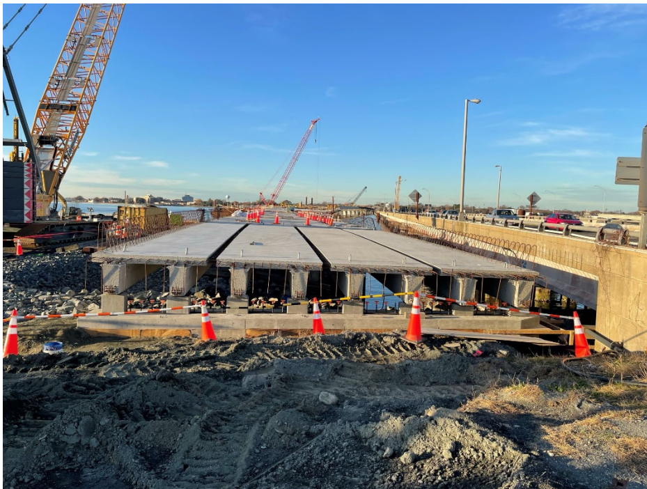
◀ North Eastbound MOT Trestle Beam and deck completion
